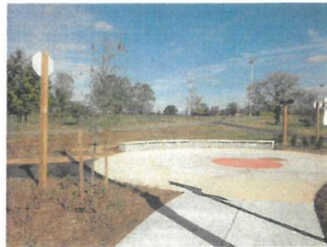
L/KLA was responsible for developing the design character of all structures along the trail in a manner that is sensitive to the natural context of the Anacostia River and Kenilworth Aquatic Gardens
