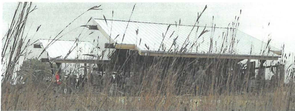
Nachusa Visitor Use Center, construction almost completed, October 2017.
