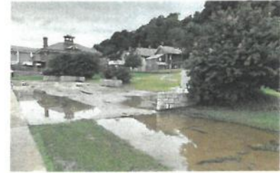
Frequent nuisance flooding at the waterfront
