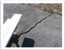
Access issue: Access path is damaged with cracks larger than  $\frac{1}{4}$
