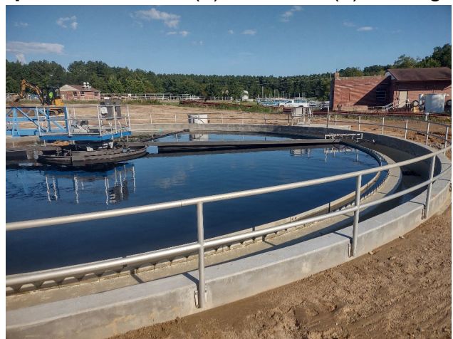
The completed Secondary Clarifier at Marlay-Taylor WRF
