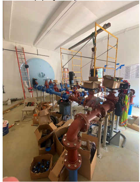
The newly constructed King Kennedy new pipe gallery.
