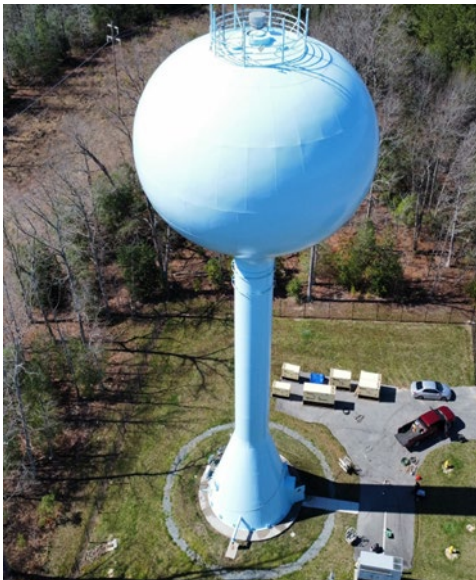
An aerial view of the Hollywood water tower after cleaning and pressure washing.
