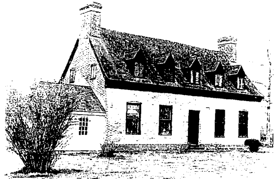
Figure 2. Ocean Hall (c. 1703) was one of the first buildings in St. Mary's County placed on the National Register of Historic Places in 1973. The lack of protection offered by this program, however, prompted a later owner to put a Maryland Historical Trust Easement on the house in 1986 to guard against future unsympathetic architectural and environmental changes. Photo by Elizabeth Hughes.
