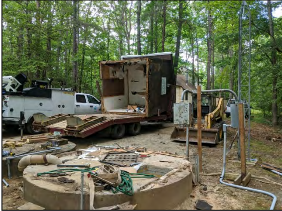
Removing the old control building at the Wildewood #1 wastewater pump station.
