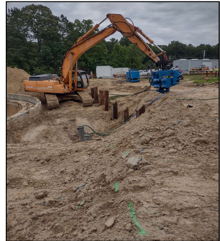
Demolition of the existing clarifier tank.
