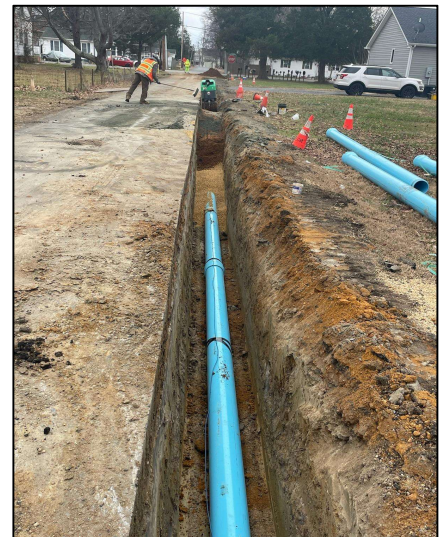
Installation of new water lines by MetCom's contractor.
