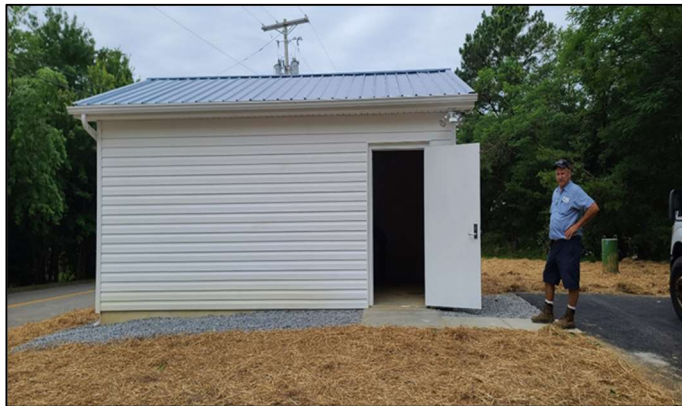
Shown above is the newly completed water station in Town Creek, which will help serve the surrounding neighborhood for years to come.
