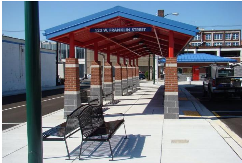
Hagerstown Transfer Center (Source: Kevin Cerrone)
